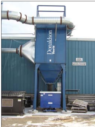
54MBTH8 at a cabinet shop on wood dust, cutting, moulding and sanding
